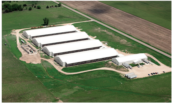
Oregon Tilth certifies these two-story henhouses with multiple tier aviary systems. Buildings have small screened porches along each side that a small fraction of birds can access. Note semi-trailers in foreground for scale of operation.
